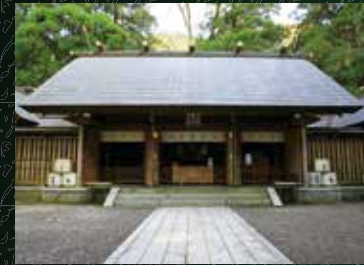
The "heavenly rock cave" from the myth of Amaterasu is the object of worship at the West main shrine building's main hall
